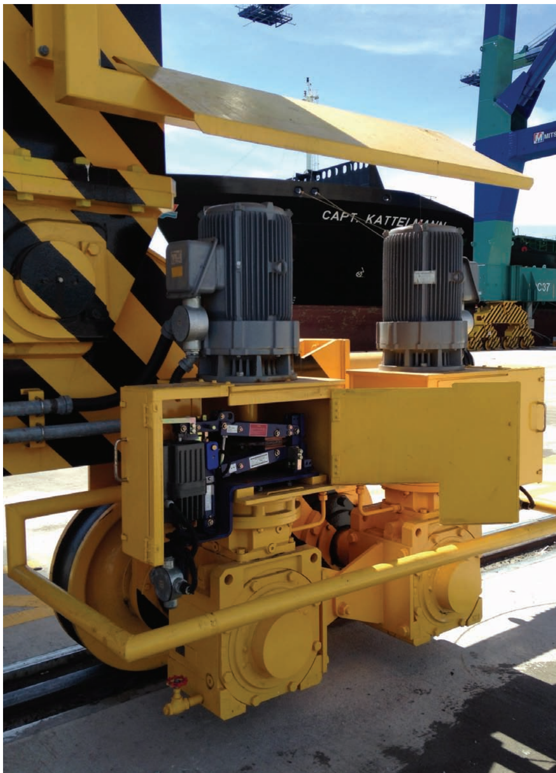
Mid-Mounted Brakes (IB30V) on 22 sets of Container crane at Westport in Malaysia
